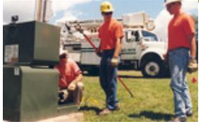
**Allow 10 feet of clear space in front of transformers.** At least once a year, our service workers open and work on the transformers while they are energized so you and your neighbors don't have to sit in the dark. To safely do that, they use an 8-foot fiberglass "hot stick" which needs about 10 feet of clear space in front of the transformer.
